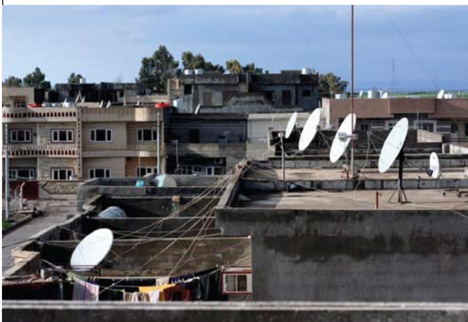
Satellite dishes are now commonplace on Iraqi rooftops
